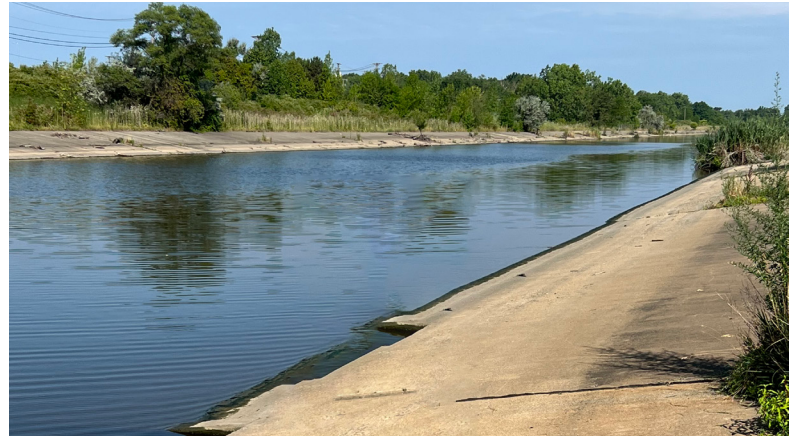
Rouge River concrete channel.
